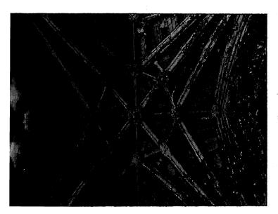
Chapter House.\* The construction of the vaults can be studied best in the cloister and the vestibule of the Chapter House, as there they are near the eye. It will be seen in the ambulatory (89) that with such a combination of four converging diagonal ribs a bay of any shape can be vaulted. In the radiating chapels (89) the vaulting problem is still more complex; for each is in plan a truncated octagon; but the problem is solved quite simply by employing seven ribs instead of four, springing
